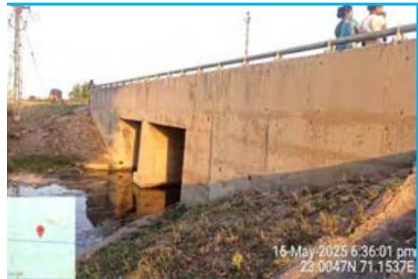
Spalling in pier at MNB 156+835
