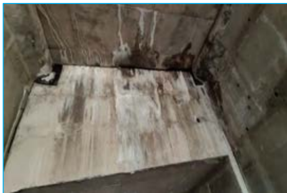
Joint leakage at MNB at Chainage 32+576
