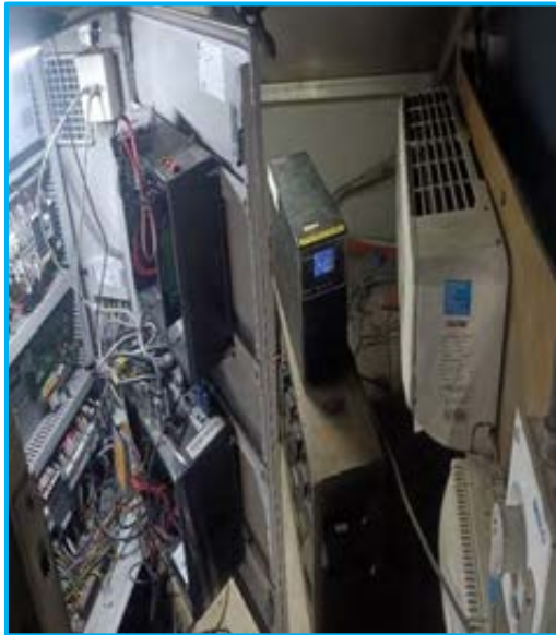
Lane Controller installation over the toll booth
