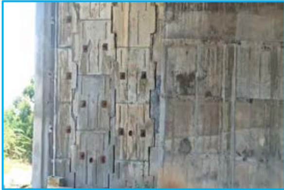
Soil nailed in RE wall
