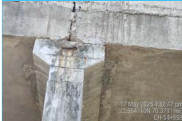
Reinforced exposed on pier at Chainage 55+223
