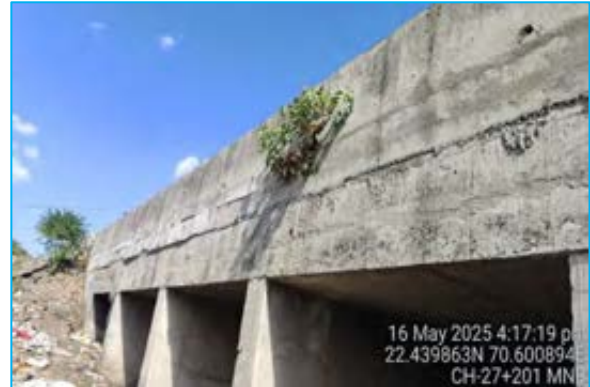
Vegetation observed on MNB at Chainage 27+201
