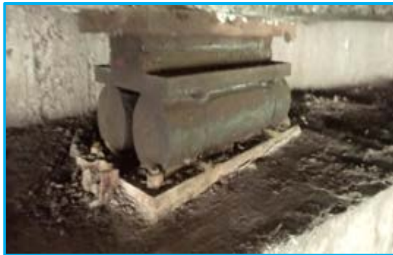
Debris and soils around the bearing area at MNB 95+930 ( Bearing at Outer Girder)
