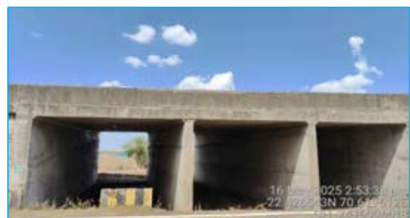
Water flow blockage observed at Chainage 18+193
