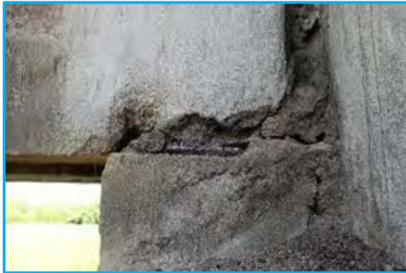
Bearing deformation at Ch.163+380
