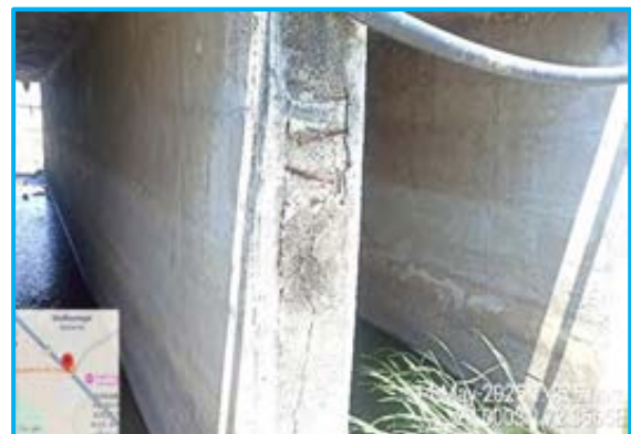
Spalling on pier at MNB Ch. 26+120
