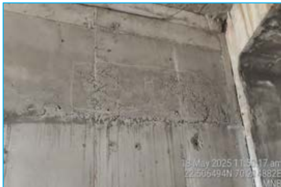
Honeycombing on pier at Chainage 73+210
