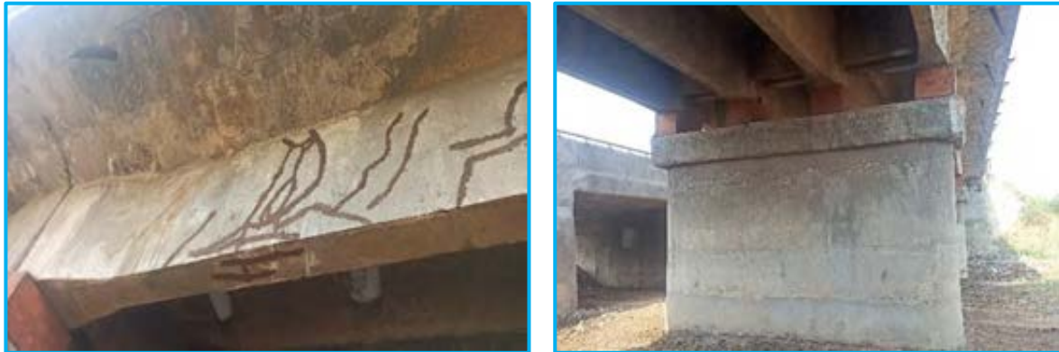
Cracked repaired at Ch. 316+115
