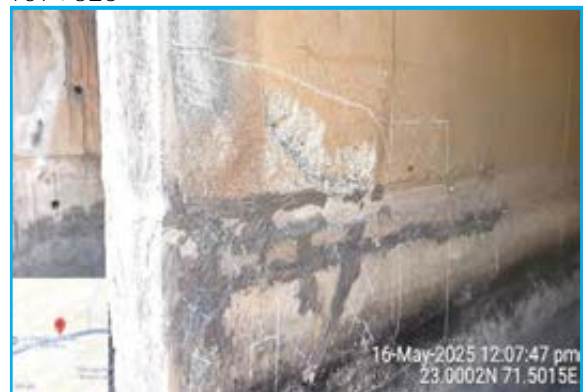
Spalling in pier at MNB Ch. 118+615
