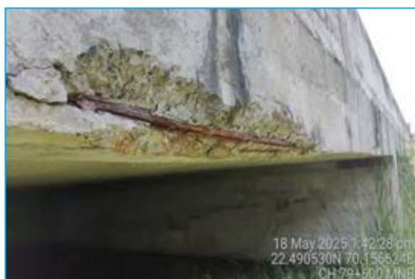
Reinforcement exposed on edge slab at Chainage 79+600
