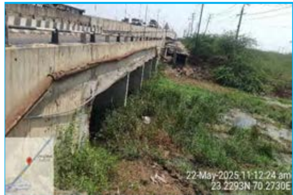
Spalling on Abutmetn Edges at MNB Ch. 334+786
