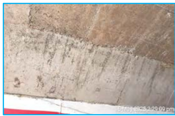
PUP at Ch. 131+535 Honey combing on soffit of deck
