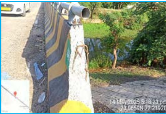
Crash barrier damaged at MNB 42+535
