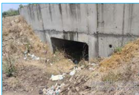
Box Culvert at Chainage 73+530
