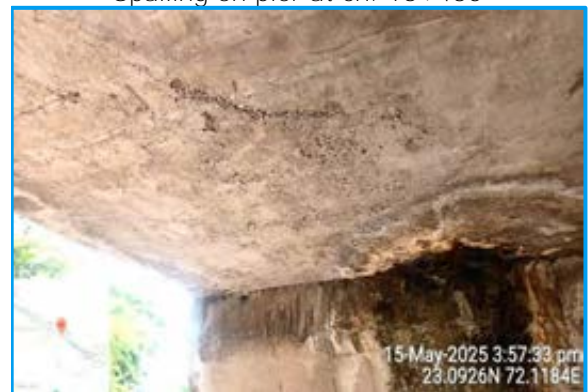
Honey combing soffit of deck slab at MNB Ch. 53+200
