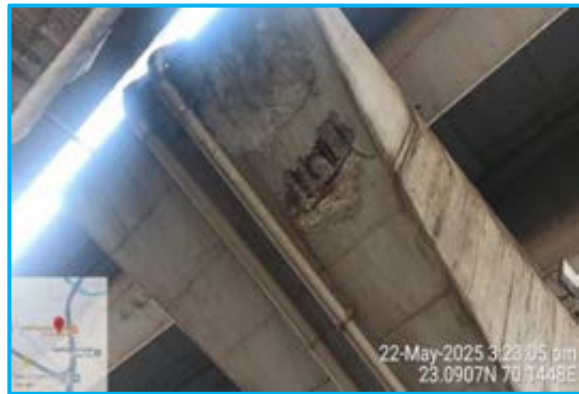
Spalling found on pier cap Flyover at 356+315
