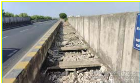
Spalling on deck slab at Chainage 83+550
