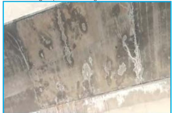
Multiple cracks in deck slab at Ch. 149+016
