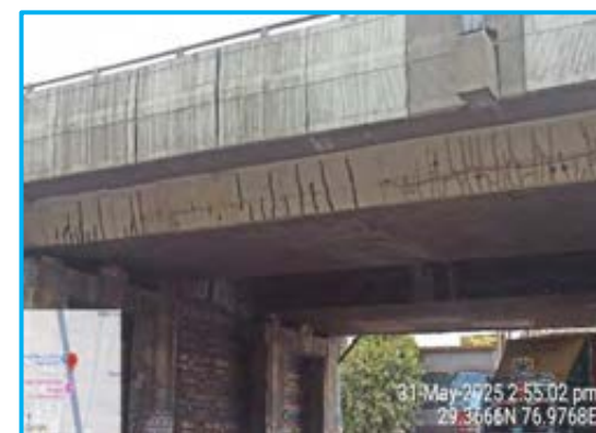
Repaired cracks on slab
