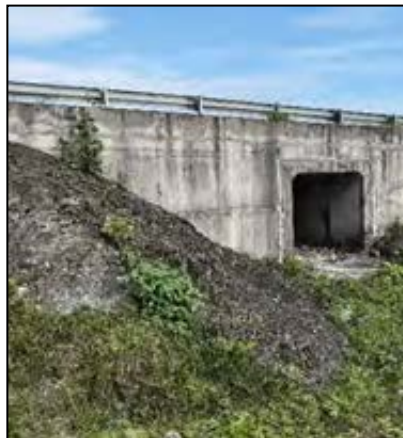
Box Culvert at Km 10+548
