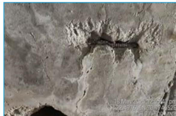
Reinforcement exposed on slab at Chainage 77+500
