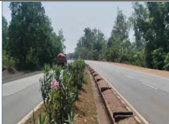
A view of the Median Drains at km 97.000-Median
