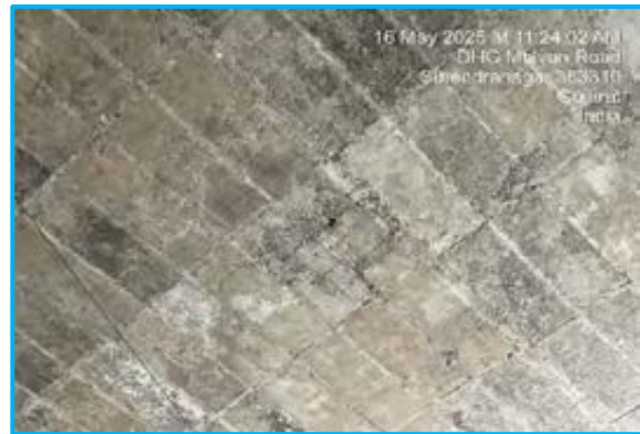
VUP at Ch. 114+900 Honey combing on soffit of deck
