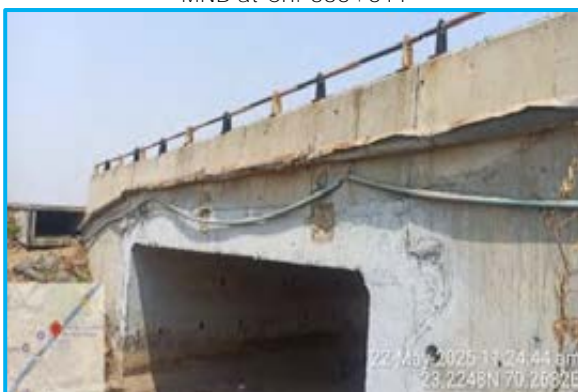
Minor spalling at edges of deck slab at MNB Ch. 335+511
