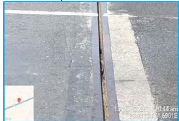
Rubber sealing damaged at MNB ch. 98+440
