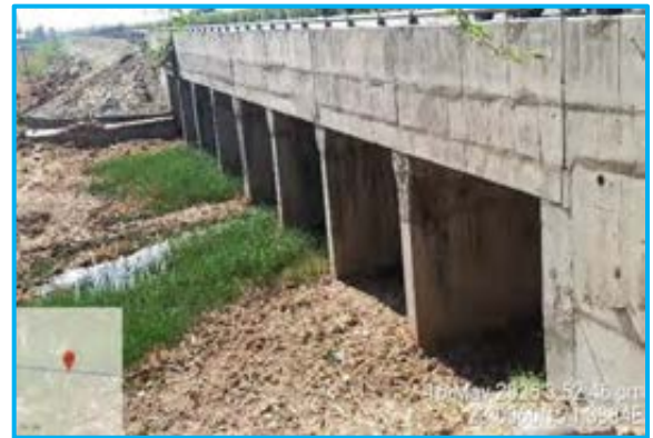
Spalling in pier at MNB 137+120
