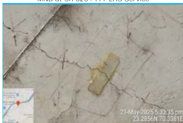
Crack in deck slab at MNB Ch. 325+317 (LHS Service)
