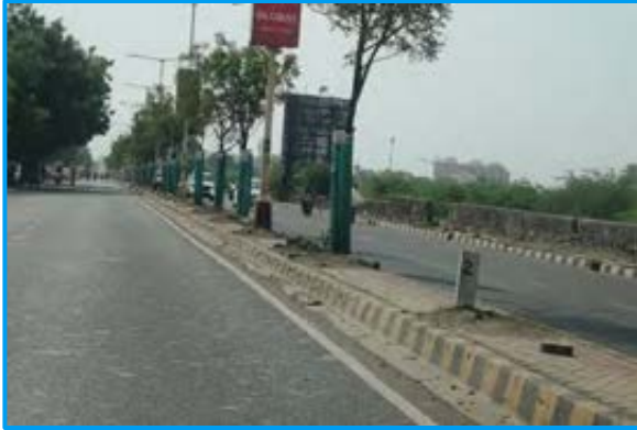
Figure 5-13: Kilometre Stones & Hectometre Stones
