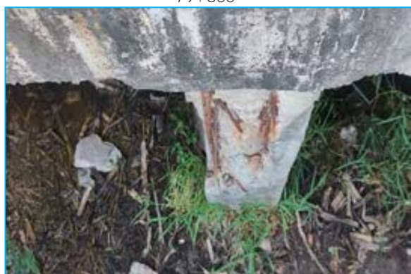
Reinforcement exposed on pier at Chainage 82+300
