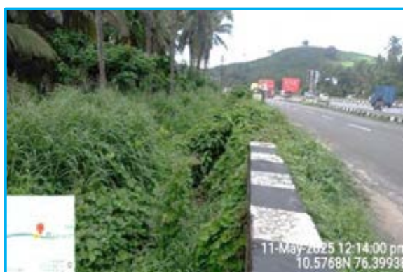
HPC at Ch. 245+807 Covered with Vegetation
