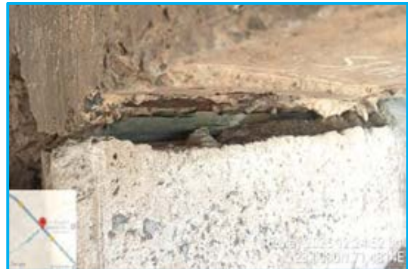
Bearing deformation at Ch.121+146 LHS
