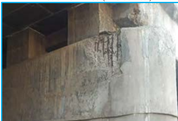
Spalling on pier cap at MNB Ch. 327+935 ( LHS)
