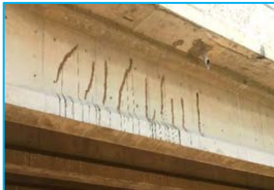
Repaired cracks at Ch. 187+730
