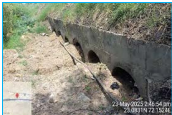
HPC at Ch.49+425 blocked with mud
