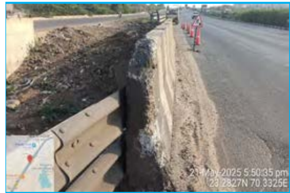
Damaged Crash barrier at MNB Ch.326+224 (LHS)
