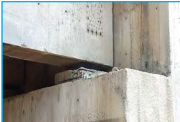
Damaged pedestal at MNB at Ch. 98+440
