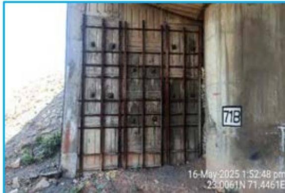
Steel framed with nailed on RE wall at Ch. 125+100
