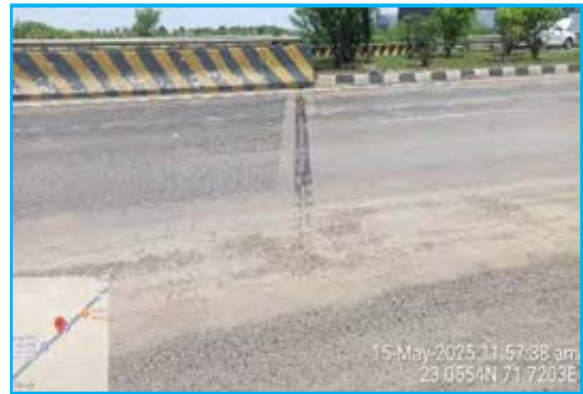
Derbis in expansion joint at Ch. 94+935
