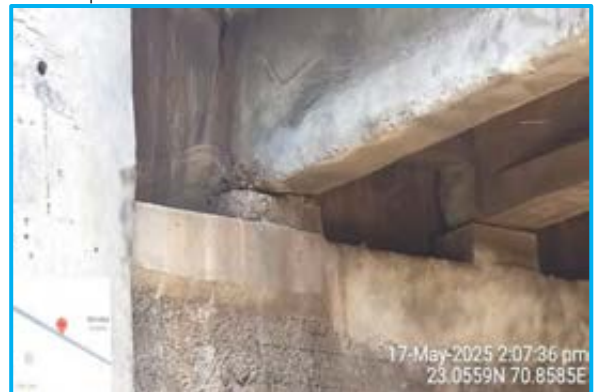
Damaged pedestal at Ch. 187+730
