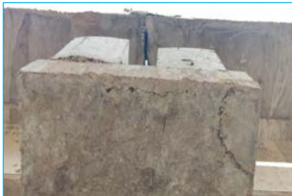
Edge Crack on Pier Cap at Chainage 89+100
