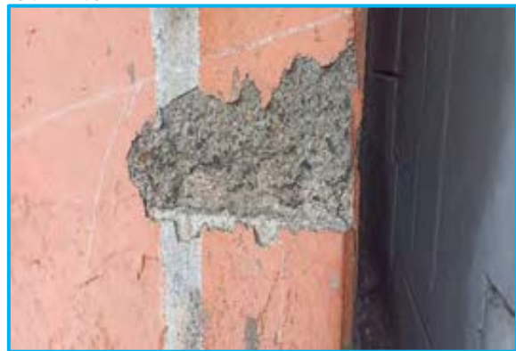
Spalling at bottom of Abutment wall at Flyover Ch.341+740
