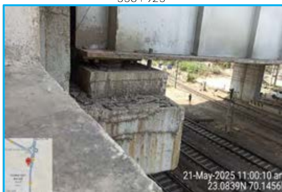
Paintless bearings ROB at Ch. 356+925
