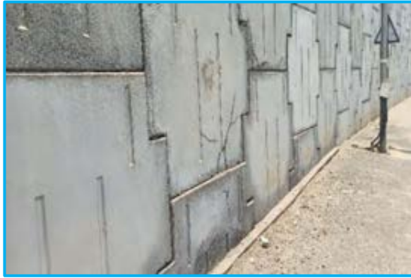
Panel cracked Flyover at Ch.341+700
