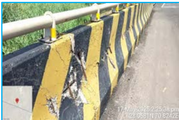
Spalling in crash barrier at Ch. 191+600
