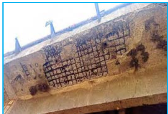
Spalling in slab at Ch. 349+498 (LHS)
