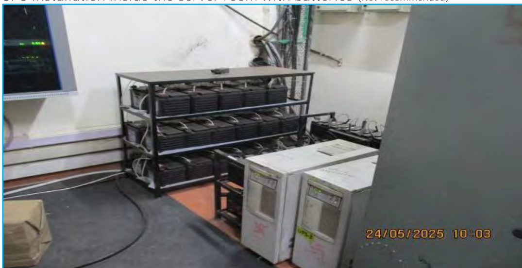
UPS installation inside the server room with batteries (Not recommended)
