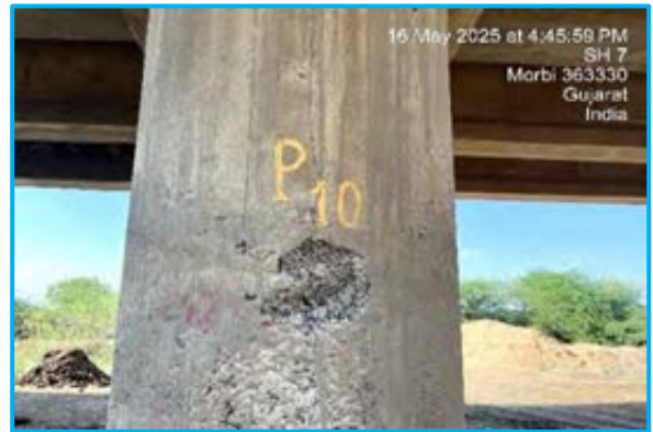
Disintegration on pier At Ch 145+824
