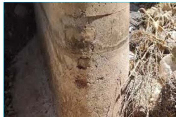
Spalling on pier at Chainage 71+120
