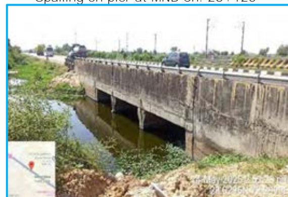
Water logging around the MNB at Ch. 32+950
