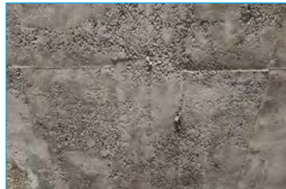
Honeycombing on slab at Chainage 74+410
