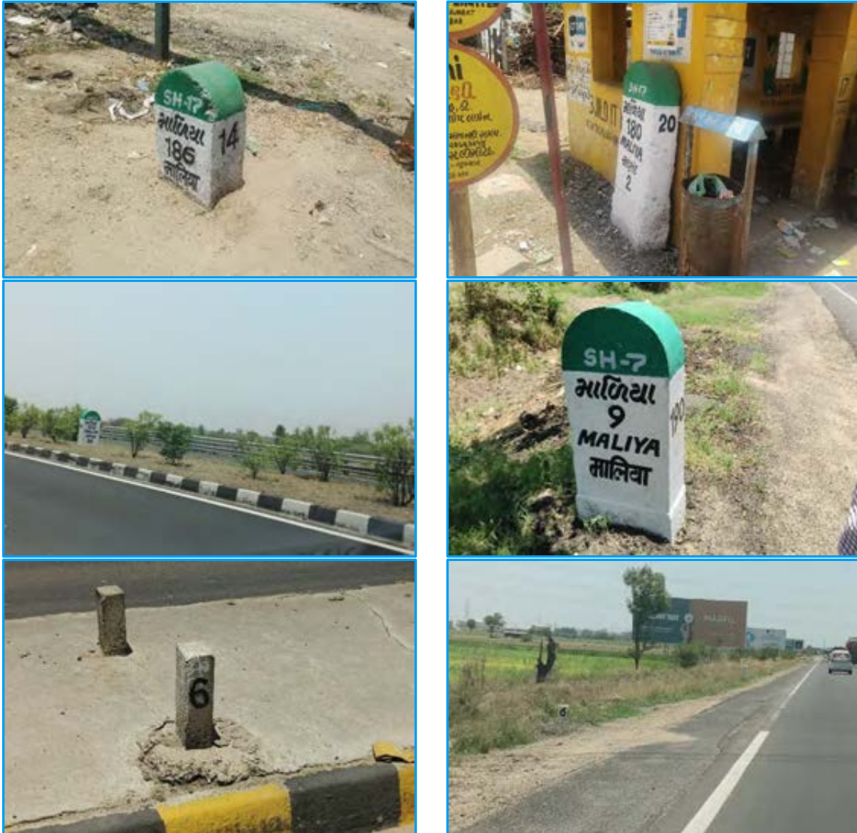
Figure 5-13: Kilometre Stones & Hectometre Stones
