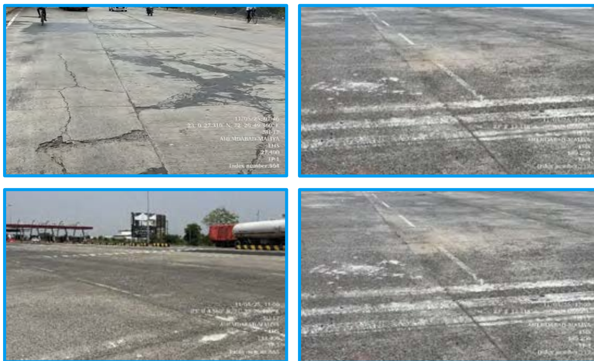
Figure 9-6: Investigation Photographs- Rigid Pavement (Toll Plaza)
