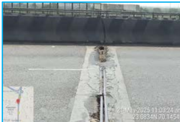
Strip seal expansion damaged at RHS ROB CH. 356+925
