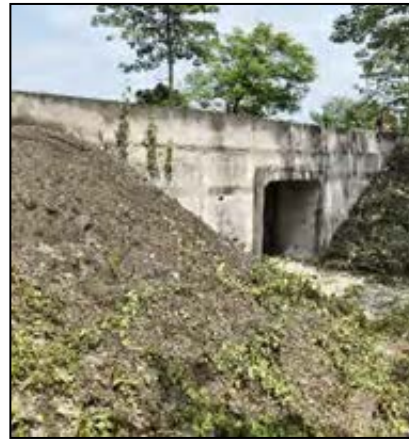
Box Culvert at Km 3+818
