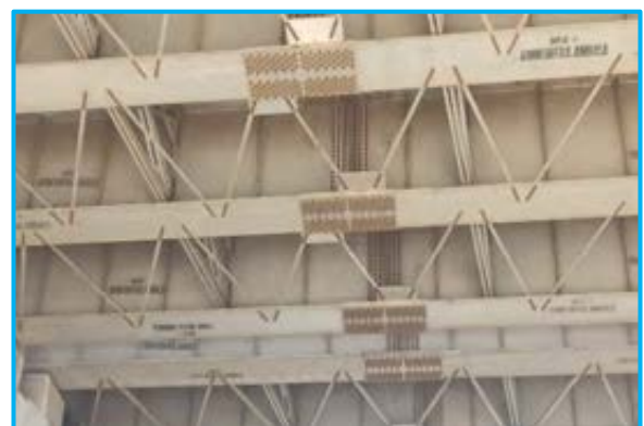
Minor corrosion on bolts at ROB Ch. 356+925
