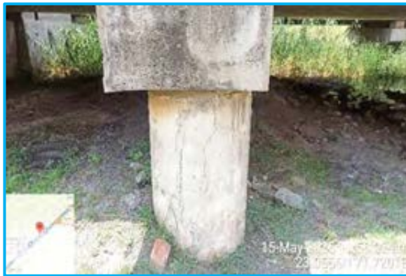
Vertical cracks in pier at MNB 94+935
