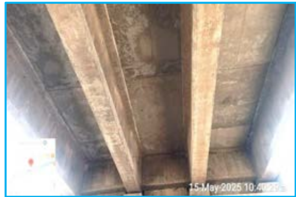
Multiple cracks in slab at Ch. 103+252
