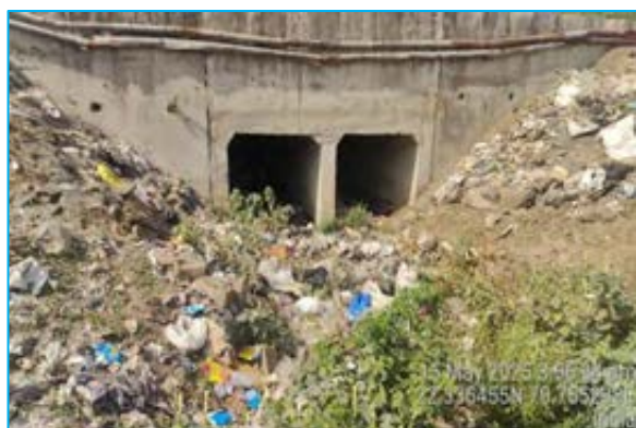
Box Culvert at Chainage 6+120
