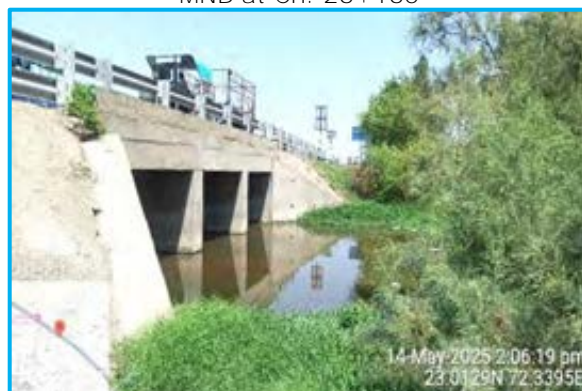
Water logging around the MNB at Ch. 28+400
