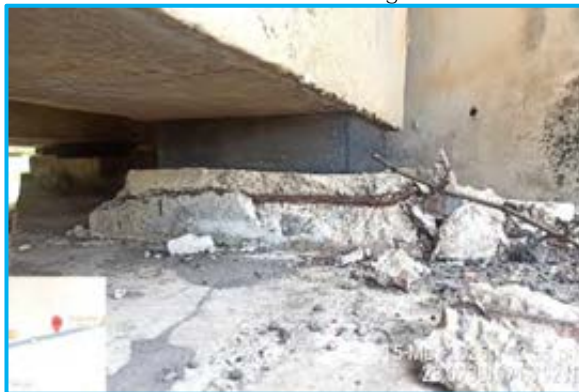
Damaged pedestal at MNB 87+200
