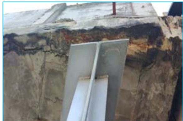
Spalling on deck slab at Chainage 83+550
