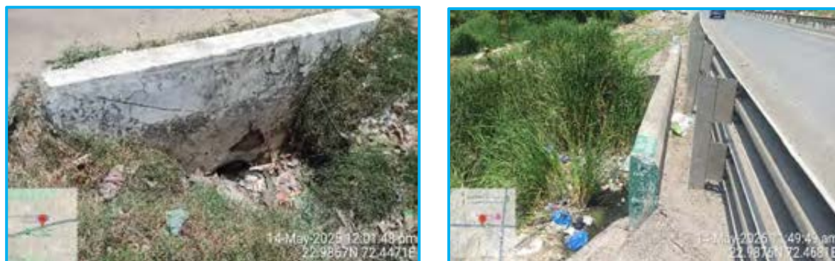
HPC Blocked with debris and mud at Ch. 16+120
