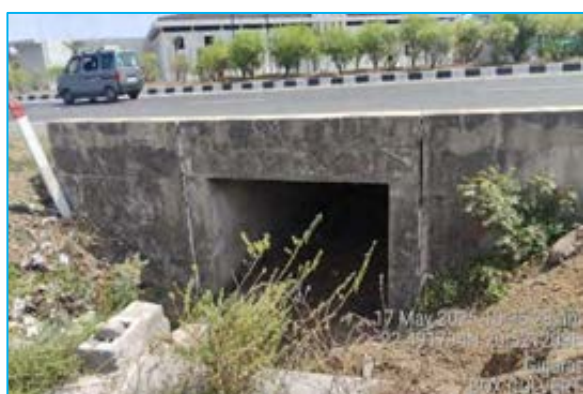
Box Culvert at Chainage 37+680
