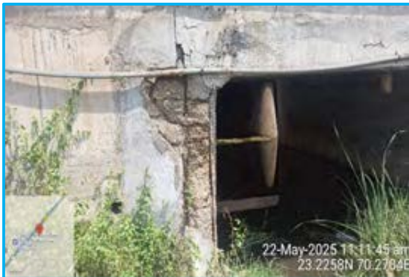
Spalling on Abutmetn Edges at MNB Ch. 334+786
