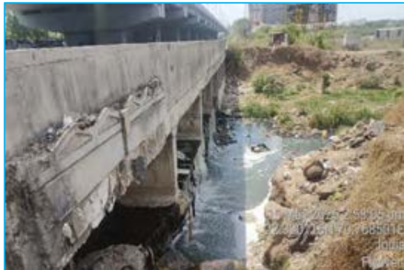
Bottom Scouring at Chainage 4+632
