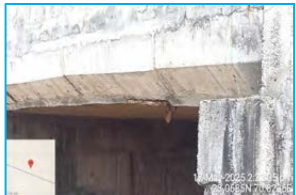
Rusted drainage spout at Ch.191+600
