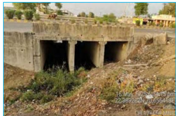
Water flow blockage observed at Chainage 18+193
