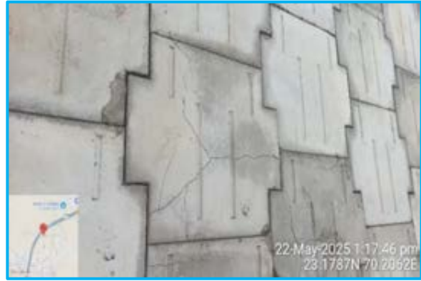
Panel cracked at Ch.344+180
