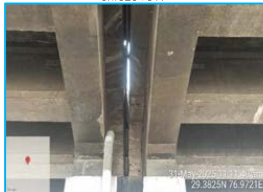
Rubber silling dmaged at expansion joint E-4
