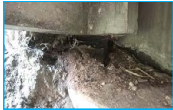
Debris and soils around the bearing area at MNB 95+930 ( Bearing at Outer Girder)
