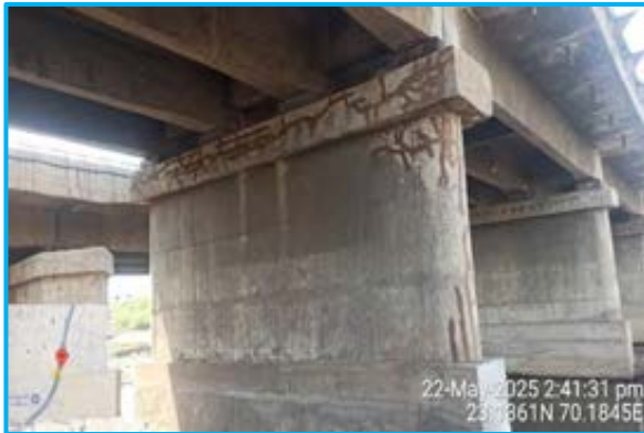
Cracked repaired at MJB Ch. 349+498 (LHS)
