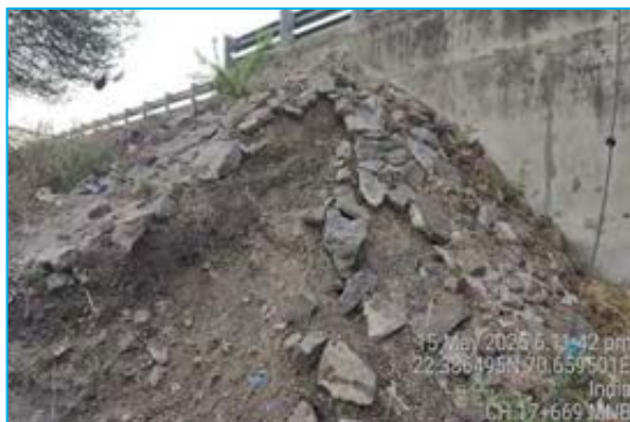
Stone Pitching damage at Chainage 17+669
