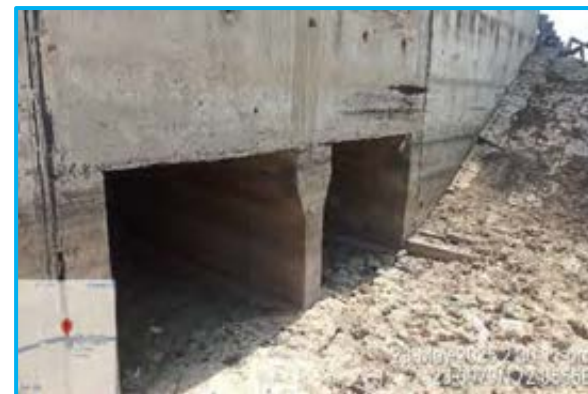
Slab Culvert at Ch. 59+780
