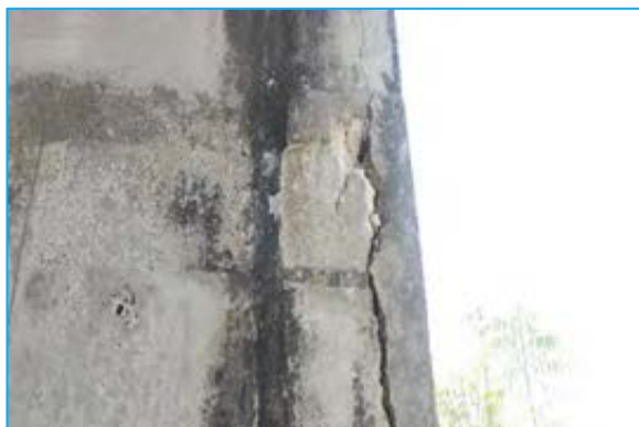
Crack on pier at Chainage 74+680
