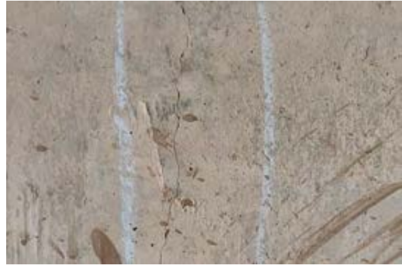
Vertical Crack at Chainage 70+800
