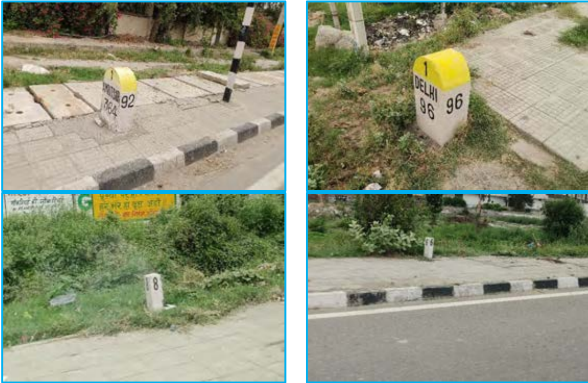
Figure 5-15: Kilometre Stones & Hectometre Stones
