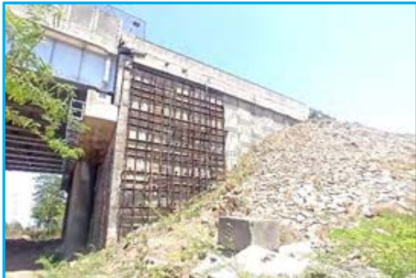
Steel framed with nailed on RE wall at Ch. 125+100
