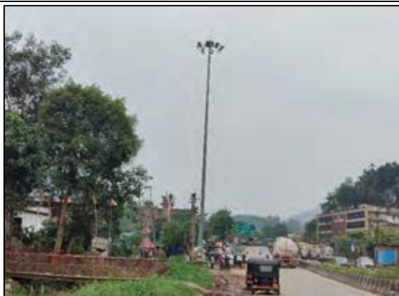
A view of High mast lighting at km 0+000 LHS
