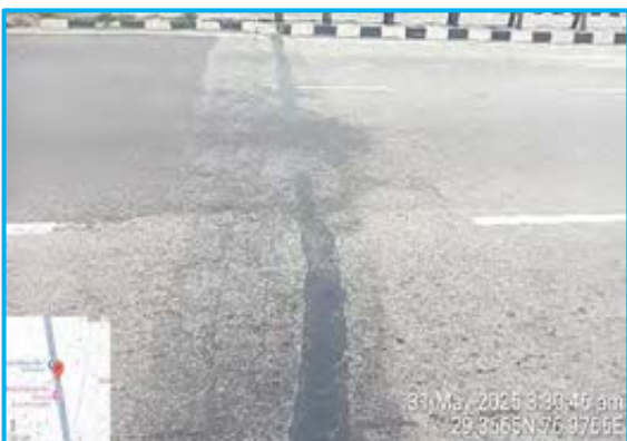
Covered expansion joint (E-1) at VUP Ch.
