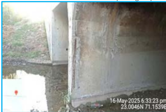
Spalling in pier at MNB 156+835
