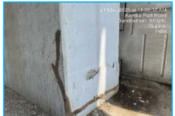
Spalling at bottom of Abutment A-1 Ch. 356+925
