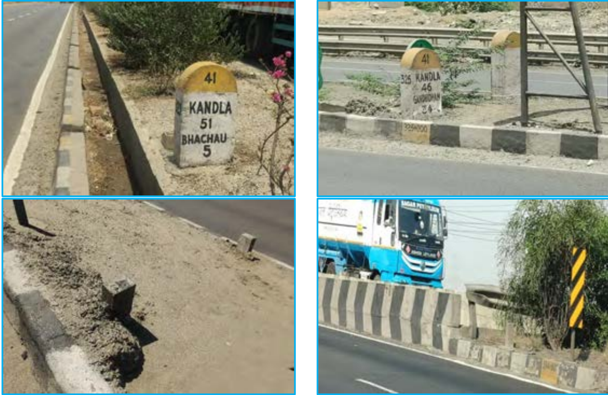
Figure 5-16: Kilometre Stones & Hectometre Stones
