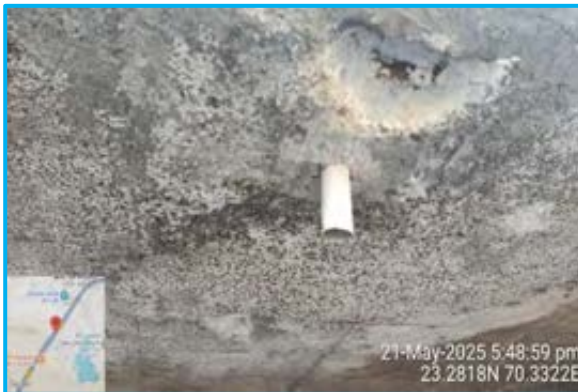
Exposed aggregates of deck slab at Ch. 326+224
