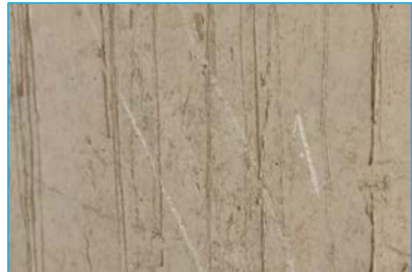
Crack on wall at MNB at Chainage 29+789
