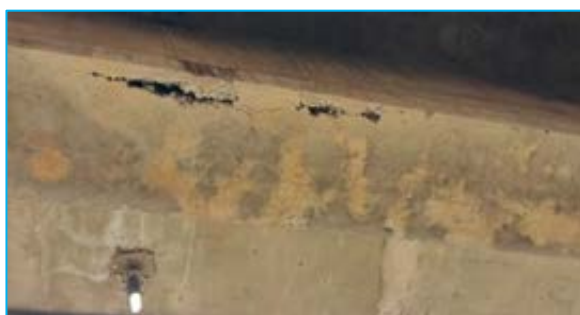
Stone Pitching damage at Chainage 17+669
