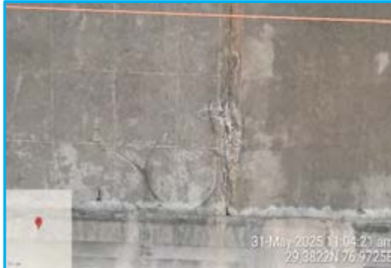
Leaching at joint Flyover at Ch. 325+317
