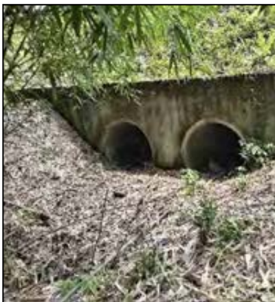
Pipe Culvert at Km 7+260
