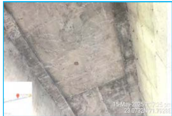
Multiple cracks in deck slab 87+200
