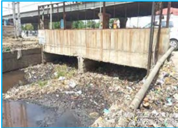
MNB at Ch. 91+410 Blocked with debris and garbage accumulation
