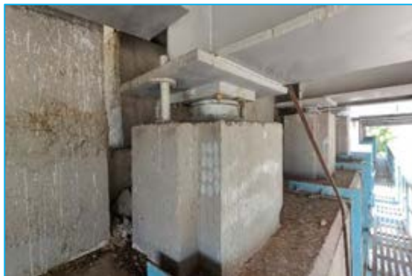
Bearing in Good Condition at Chainage 24+400
