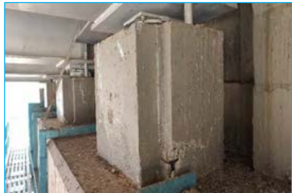
Wide multiple cracks observed on pedestal at Chainage 24+400
