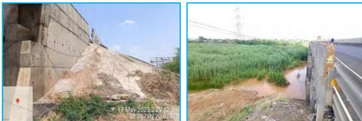
Vegetation around the structure at Ch. 191+600
