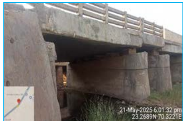
Spalling on pier cap at MNB Ch. 327+935 ( LHS)
