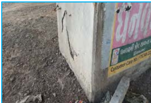
Spalling in pier at Ch. 324+035
