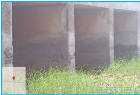
Spalling in pier at MNB 137+120
