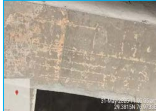
Honey combing on diaphragm at flyover Ch.325+317
