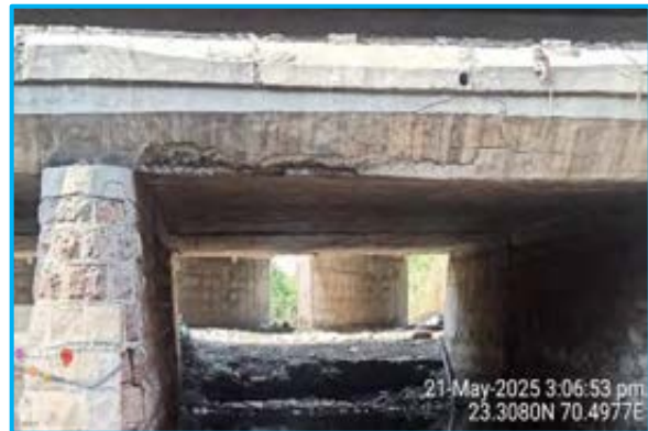
Spalling in deck slab edges MNB at Ch.308+130
