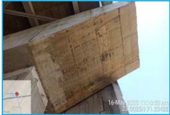
Scaling on concrete at Abutment RHS 116+300
