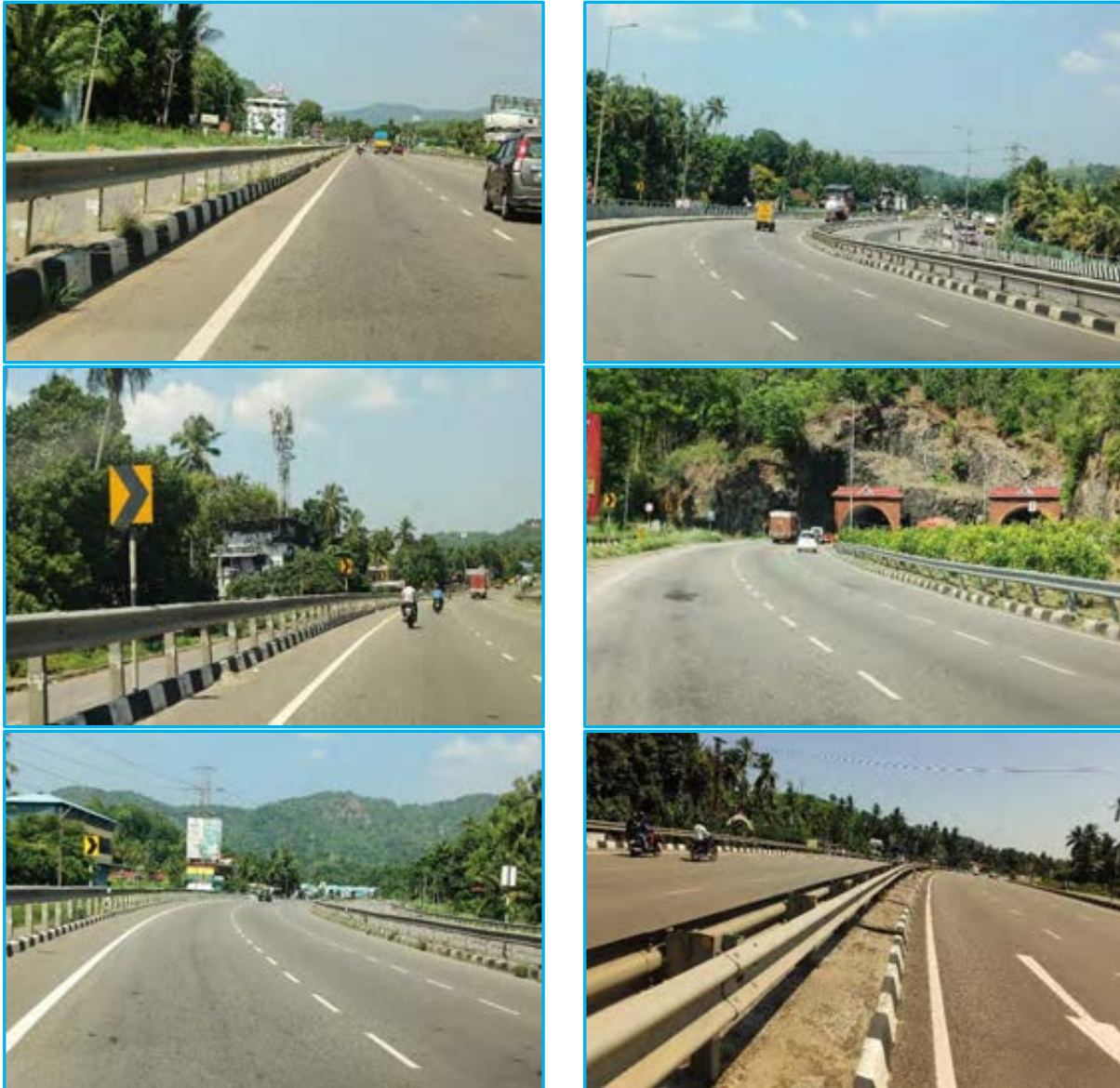
Figure 5-11: Metal Beam Crash Barriers
