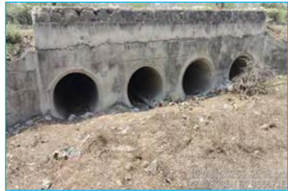
Pipe Culvert at Chainage 119+100
