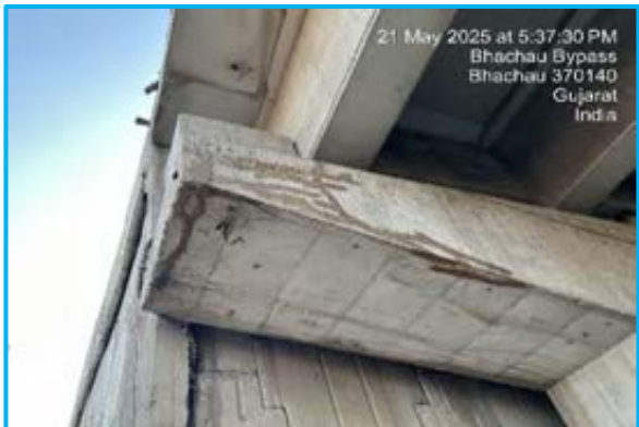
Crack repaired on abutment Cap VUP at Ch. 325+568
