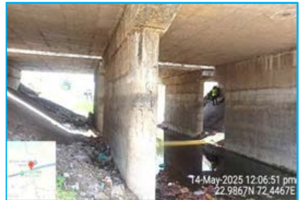
Spalling on pier at ch. 16+430
