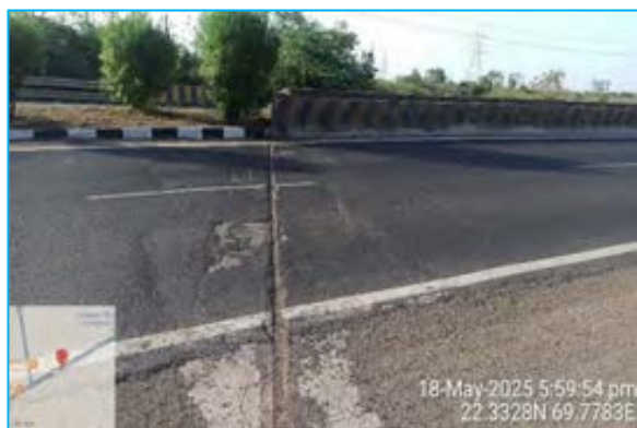
Clogged expansion joint at Chainage 128+690
