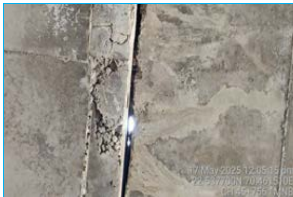
Joint leakage at MNB at Chainage 32+576
