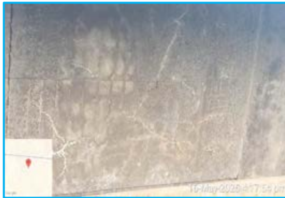
Multiple cracks in soffit of slab at Ch. 145+824
