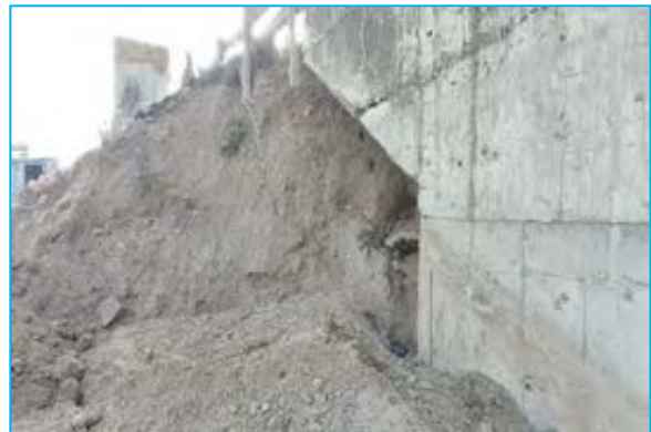
Heaving Observed near Abutment of a Major Bridge at Chainage 91+880
