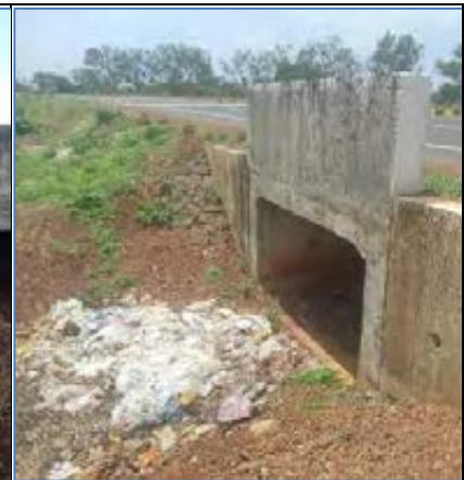
Box Culvert at Km 415+490
