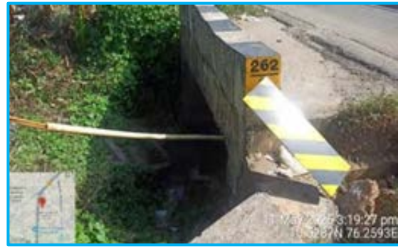
Hazard marker damaged at Box Cul. 262+942
