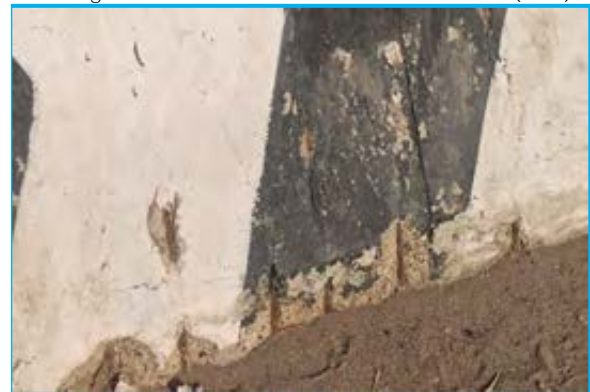
Spalling in crash barrier at MNB Ch. 326+224
