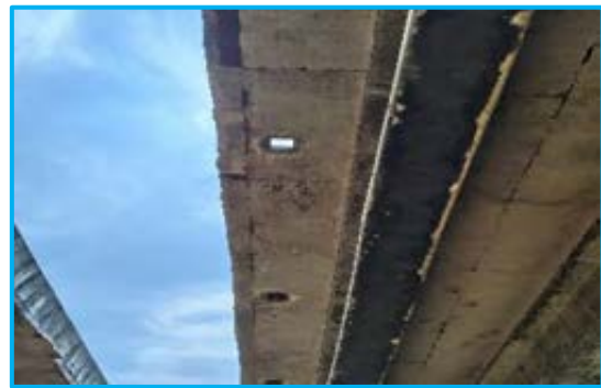
Missing Drainage Spout at Flyover 236+744
