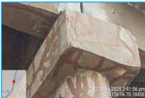
Cracked repaired at MJB Ch. 349+498 (LHS)
