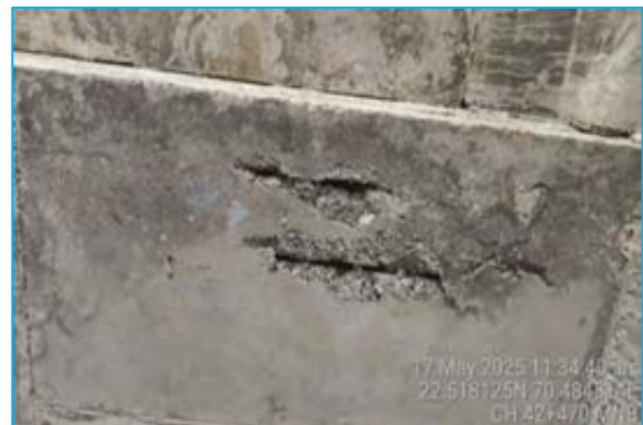
Reinforcement Exposed at chainage 42+470
