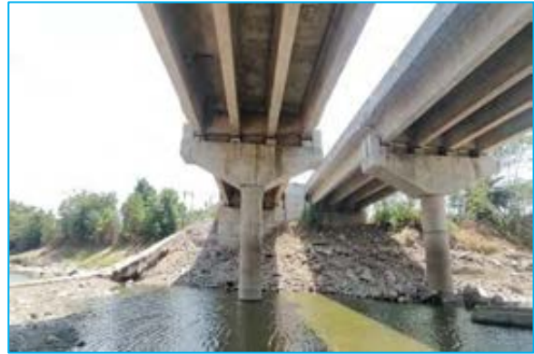
Stone Pitching damaged at Chainage 80+650
